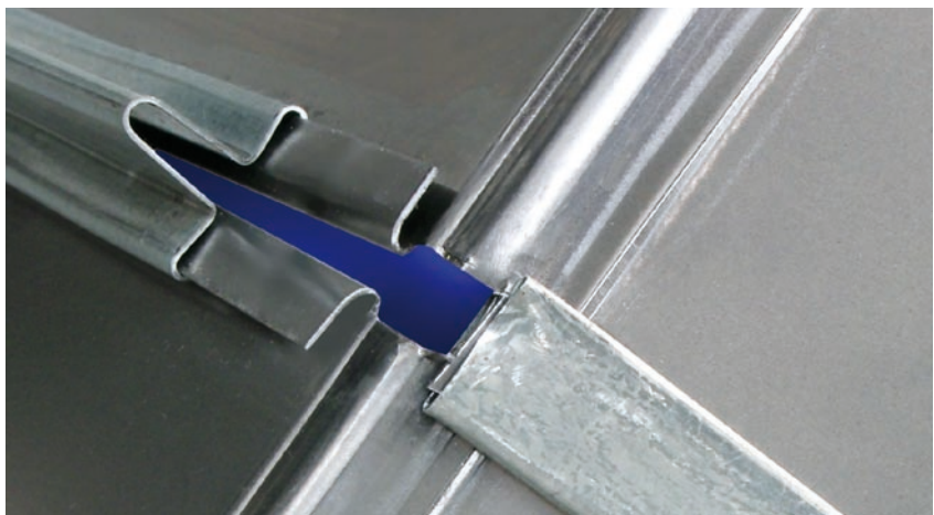
Duct connection with Suspension Drive Cleat and S-Cleat
